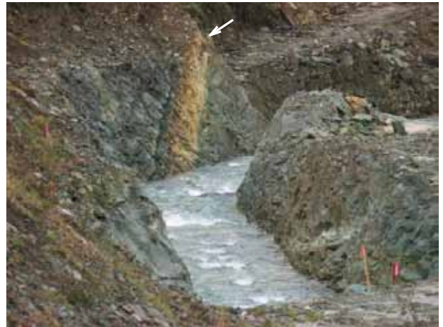
Photo 1. 市野々原地区地すべりの捷水路の河道掘削面に現れた古い断層。 An old fault observed on the bank of cut-off channel at the foot of Ichinohara landslide.
