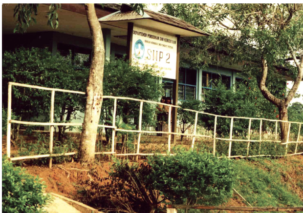
Photo. 9. A junior high school fence made with Peronema canescens poles in the Pasir region.
