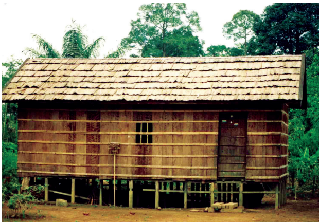
Photo. 8. A house covered with strips of Peronema canescens bark in the Pasir region.
