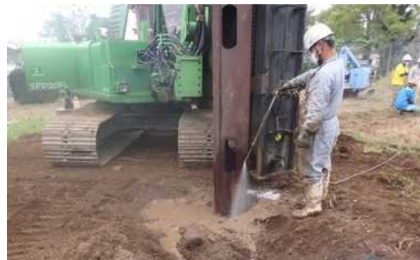
Photo 1 Excavation of a cylindrical pile.
